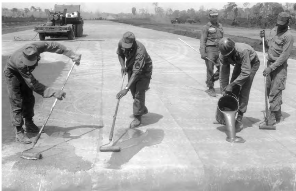
Work crews apply a nonskid compound to Duc Lap airstrip.
